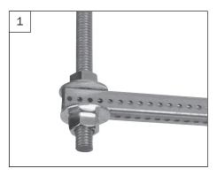
Locate holes on bracket and secure bracket to %" threaded rod using washers and %" nuts. If desired, hardware can be installed both above and below bracket. Install double nut if specified.
